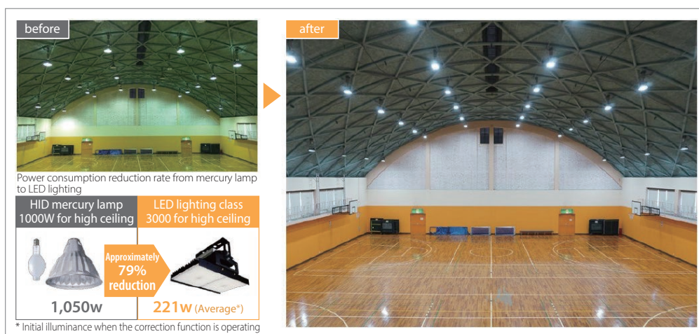
Example of LEDs at the Works: Upgrading the lighting of the gym at the Works
