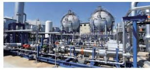
Calorific value adjustment system at Ogishima Natural Gas Supply Co., Ltd
