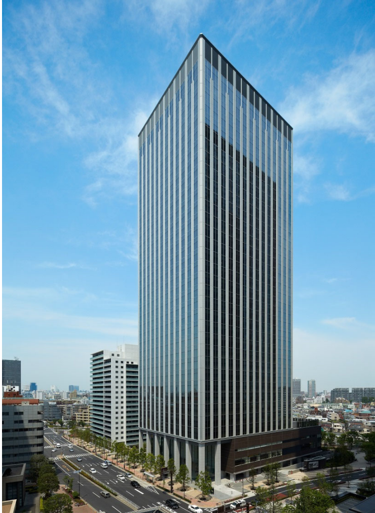
(Reference) Exterior of Shinjuku Front Tower
