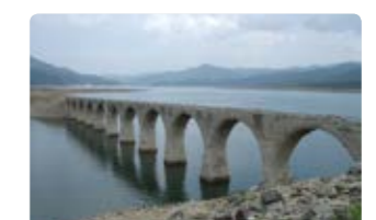
Mine cart experiences to promote tourism at a concrete arch railway bridge
