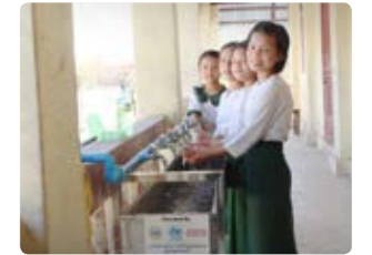
Children washing their hands at a water supply facility installed at a school (Myanmar)
