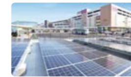
Solar panel installation
