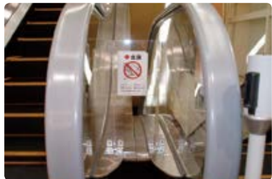
A safety measures for escalators
