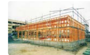
A Ministop store under construction
