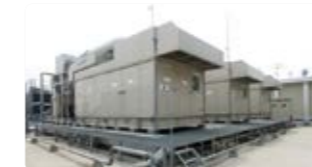
Aeon's private power generators
