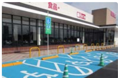
Parking lot guardrails
