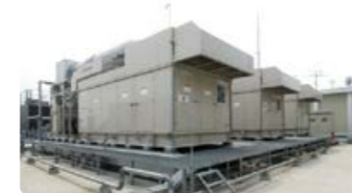
Aeon's private power generators
