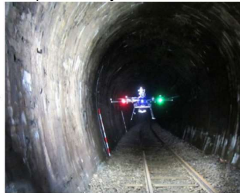
Future Inspection by drone
