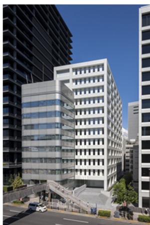
Exterior (distant view) KT Building
