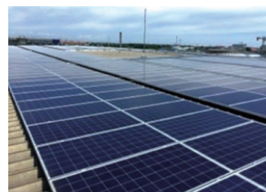
Solar panels installed on a roof
