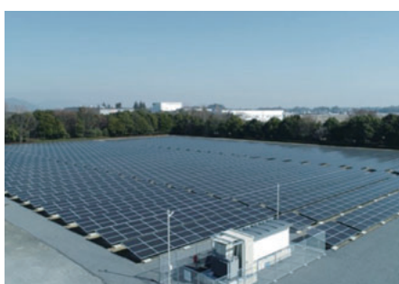
Megasolar power system at the Tatebayashi Plant (1.3 MW)
