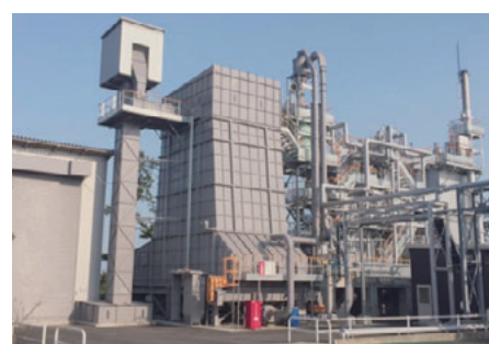
Biomass boiler at the Hokuriku Plant
