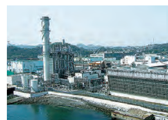
Tokyo Gas Yokosuka Power Co., Ltd.
