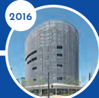
Toyosu Smart Energy Center
