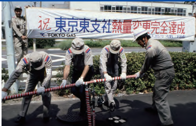
Full completion of the calorific value change in the area served by the Tokyo Higashi Branch Office
