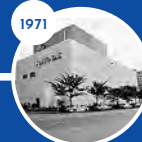
1971 The old Shinjuku District Heating and Cooling Center
