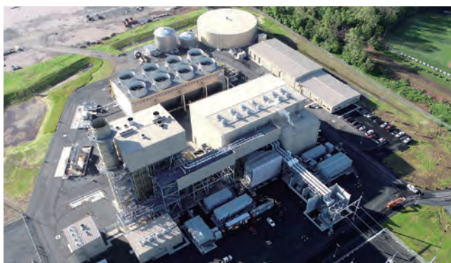
Birdsboro Power Plant
