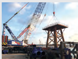
Nong Fab LNG Receiving Terminal
