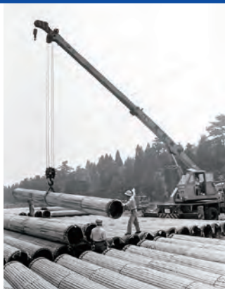
Chiba main pipeline work
