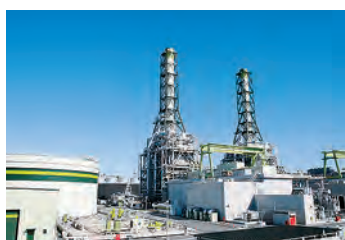
Kawasaki Natural Gas Power Generation Co., Ltd.
