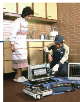
Appliance adjustment work for calorific value change at a customer's residence
