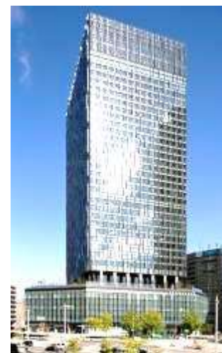
Dai Nagoya Building
