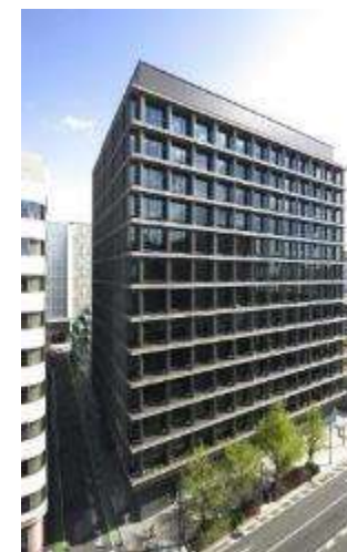
Kamiyo Hakata Chuo Building
