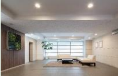
Switching to LED lights in common areas
