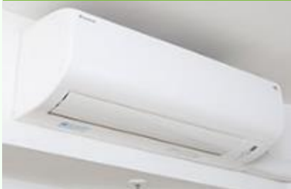
Replacing air conditioners in private areas
