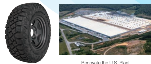
Renovate the U.S. Plant
