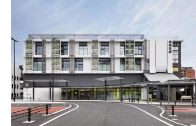
[Along JR West lines] Opening PLiCO Nishi-Akashi South Building, together with a new ticket gate and station-front plaza
