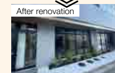
Conversion from parking to retail space in progress
