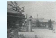
Front-view photo of the site where the two-story office was burned down in the war
