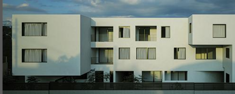
THE GRANDUO KAMIMEGURO aat+makoto yokomizo architects, Inc.
