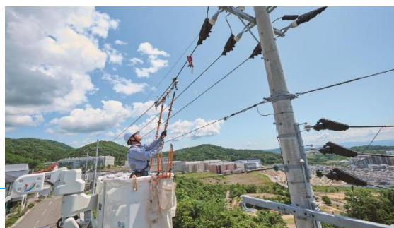
Distribution Line Inspection
