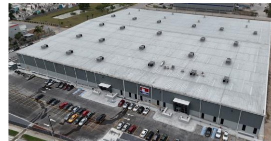
Automatic door plant in Mexico
