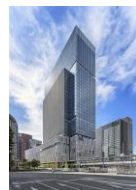
JP Tower Osaka (Opened in July 2024)
