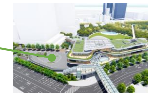
Osaka Station Umekita area
