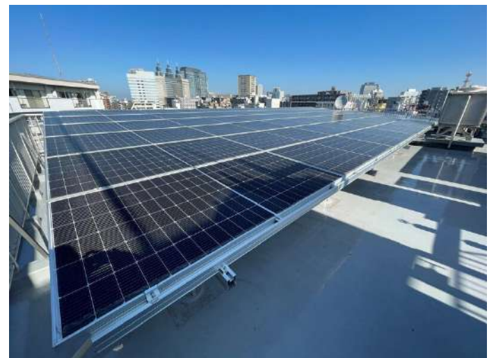
Solar panels installed on the rooftop
