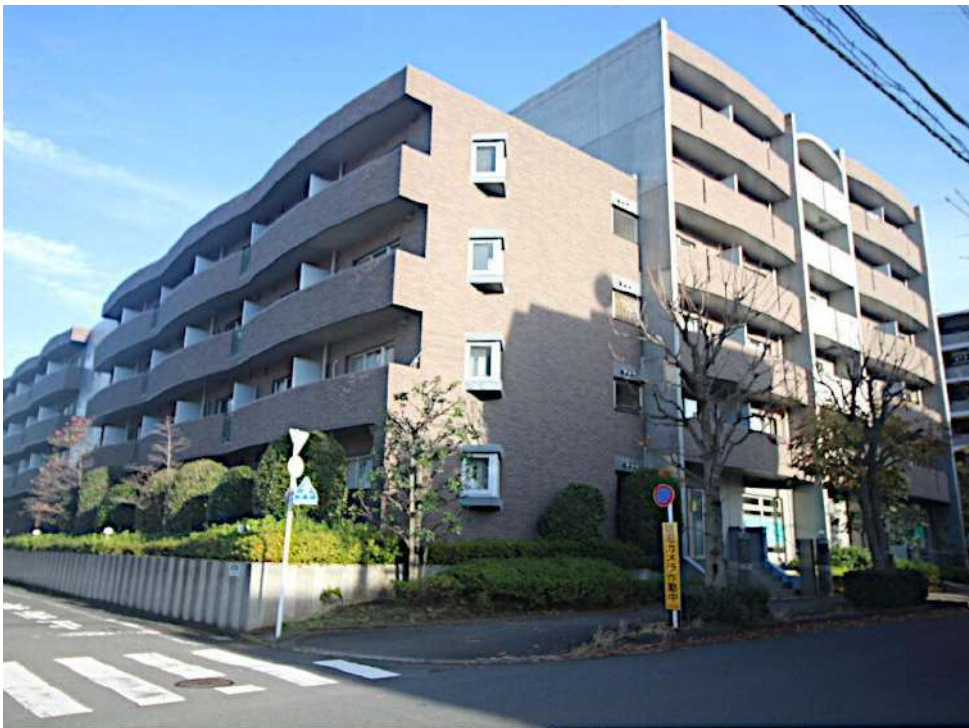
Exterior view of subject property
