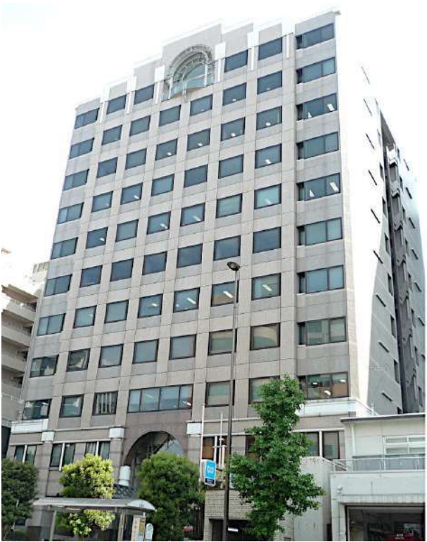
Narimasu Tosei Building
