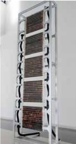
Rear door chilled water heat exchanger for data center servers
