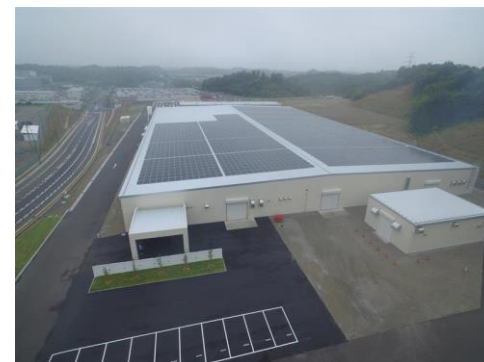
Completed new plant – exterior view
