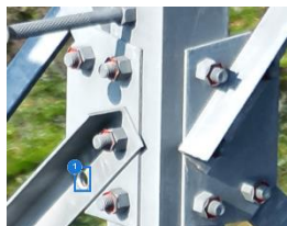
Detection of holes where bolts have fallen out
