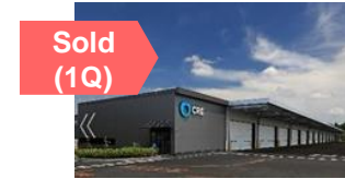
LogiSquare Narita (Chiba Prefecture) total floor area:18,022 sqm
