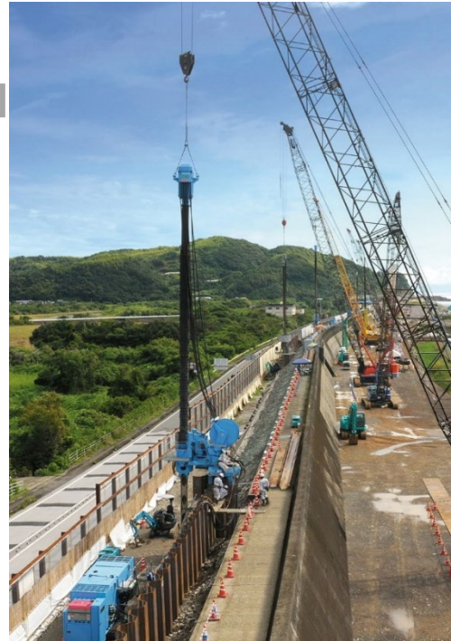
Hard Ground Press-in Method
