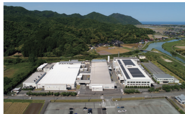
Solar panels installed at the Tottori Plant (Tottori Prefecture)
