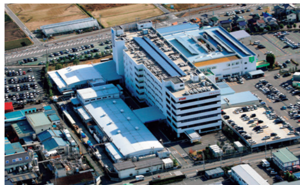
Solar panels installed at the Takasaki Plant (Gunma Prefecture)
