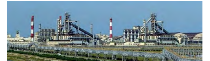
Formosa Ha Tinh Steel Corporation's integrated steelworks
