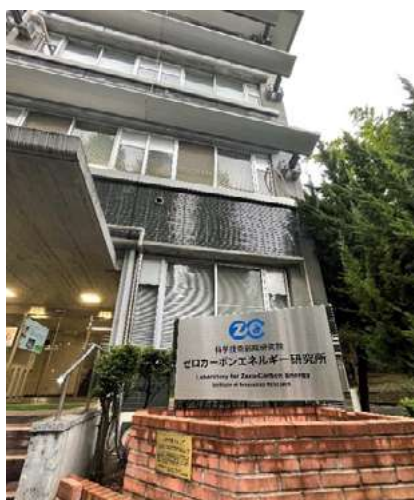
Laboratory for Zero-Carbon Energy, Institute of Innovative Research (Ookayama North No. 1 Campus)
