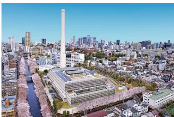
Waste-to-energy power generation plant
