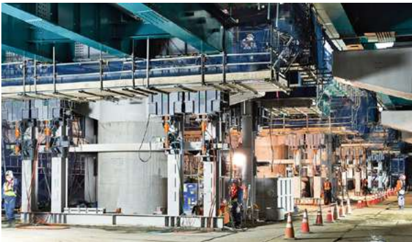
Installing a beam with the Jack-up Method
