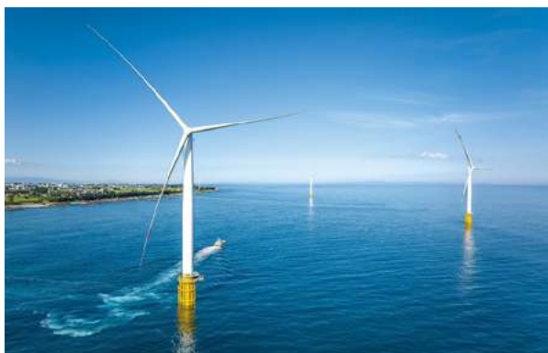
Nyuzen offshore wind power station (Photo by VENTI JAPAN, Inc.)
