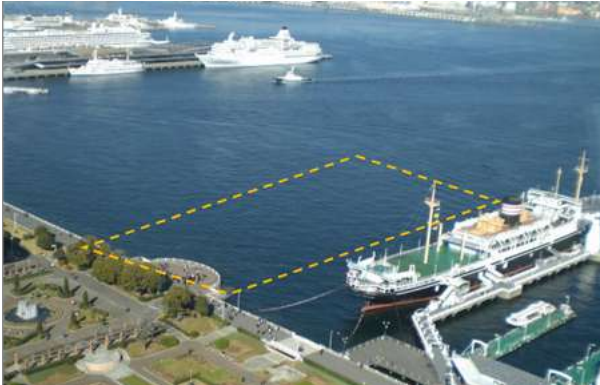
The dotted line indicates the area in which slag products are being used at Yokohama Bay (photo taken by Yokohama City)
