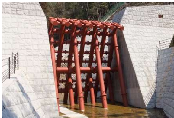
Permeable steel slit dams
