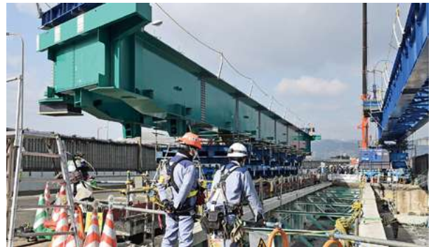
Replacing an old beam with a new one
