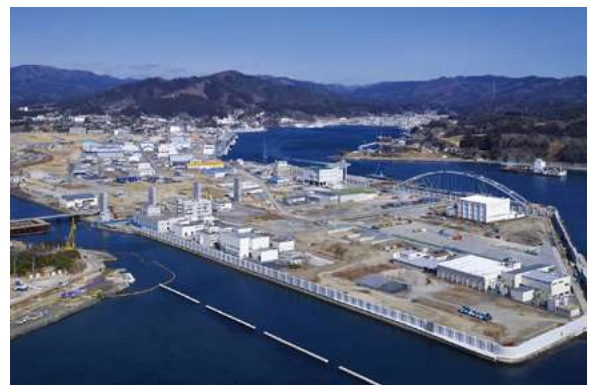
Hybrid tide embankments
