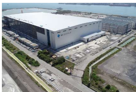
Monopile manufacturing plant during its construction (May 2023)
