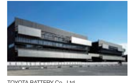
TOYOTA BATTERY Co., Ltd. Arai Plant No. 2 (Shizuoka Pref.) (air conditioning and plumbing works)
