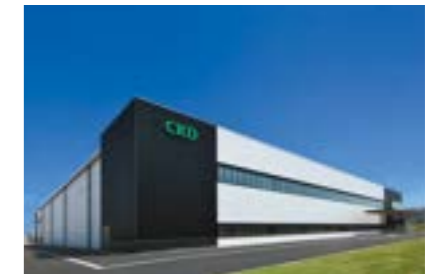
CKD Corporation Hokuriku Plant (Ishikawa Pref.) (electrical work)
