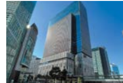
JP Tower Osaka (air conditioning and plumbing works)
