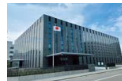
Bank of Japan Kanazawa branch (air conditioning and plumbing works)
