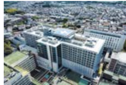
St. Marianna University Hospital Inpatient Building (Kanagawa Pref.) (air conditioning work)
