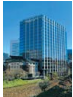
Kudan-Kaikan Terrace (Tokyo) (air conditioning work)
