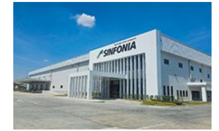
Thailand Sinfonia PH-3 Plant (air conditioning, plumbing and electrical works)
