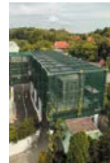
Resorts World Sentosa 2nd District Cooling Equipment Machine Room (Singapore) (electrical, air conditioning and plumbing works)
