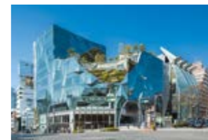
Tokyu Plaza Harajuku (Harakado) (Tokyo) (air conditioning and plumbing works) Photo: Shingo Nakajima, SS Co., Ltd.
