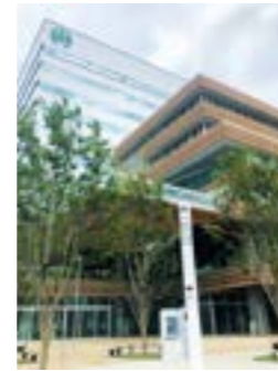
Chiba City Hall New government office (air conditioning work)
