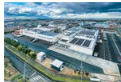
Ichimasa Kamaboko Co., Ltd. Headquarters Factory No. 2 (Niigata Pref.) (air conditioning and plumbing works)
