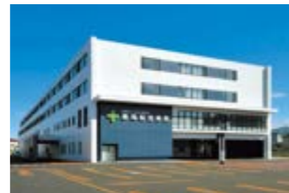
Seiwa Memorial Hospital (Hokkaido Pref.) (air conditioning and plumbing works)
