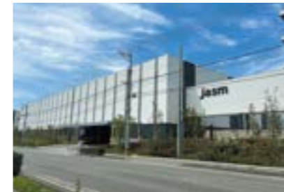
Kumamoto JASM FAB (Kumamoto Pref.) (air conditioning work)
