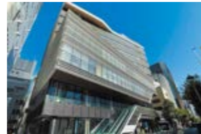
Granbell Square (Tokyo) (electrical, air conditioning and plumbing works)
