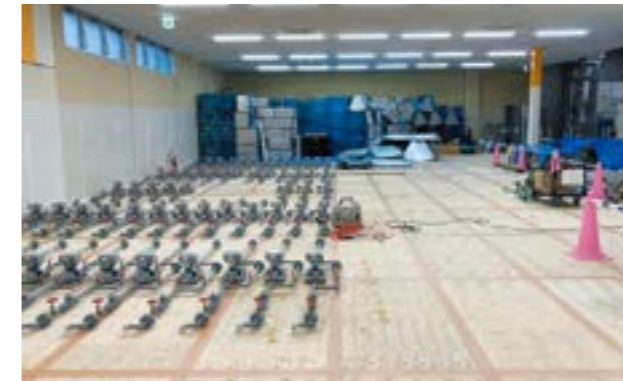
Piping unit processing
