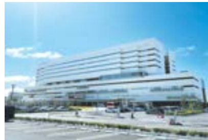
Toyota Memorial Hospital (Aichi Pref.) (electrical work)
