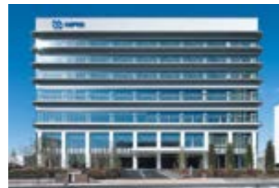
Nipro Corporation Head Office (Osaka Pref.) (air conditioning work)
