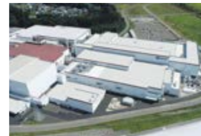
NIPRO Corporation Ohdate Factory (Akita Pref.) (air conditioning and plumbing works)
