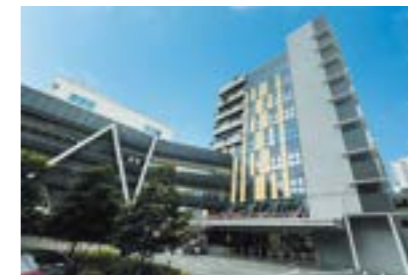
Mount Alvernia Hospital (Singapore) (air conditioning and electrical works)
