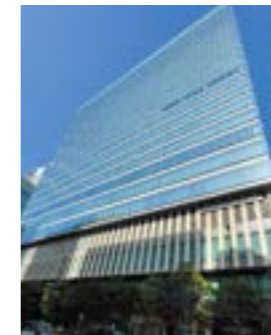
BUNKYO GARDEN GATE TOWER (Tokyo) (air conditioning and plumbing works)
