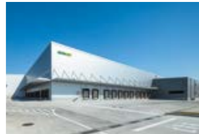
AEON Next Co., Ltd. Honda CFC (Chiba Pref.) (air conditioning and plumbing works)
