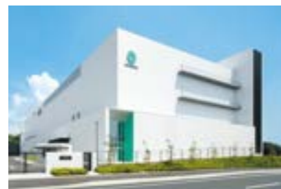
Biofermin Pharmaceutical Co., Ltd. Kobe Factory No. 2 (air conditioning and plumbing works)
