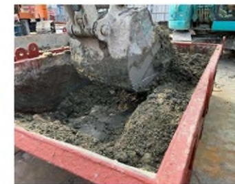
Mixing Bamboo Chips
