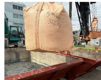
Adding Bamboo Chips to Sludge
