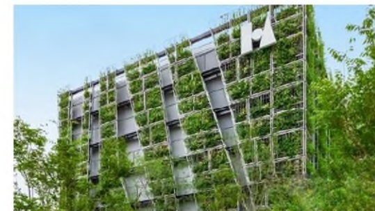
Green Wall of the Multipurpose Experiment Building
