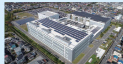
Ogaki Central Plant
