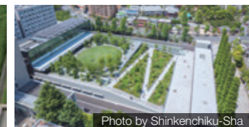
Rooftop Greening (Waseda Arena) [IBIDEN GREENTEC CO., LTD.]
