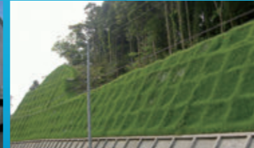
Slope greenification for environmental conservation (GT Frame Method*)
