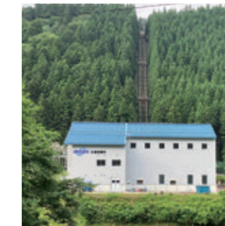
Hirose Power Plant
