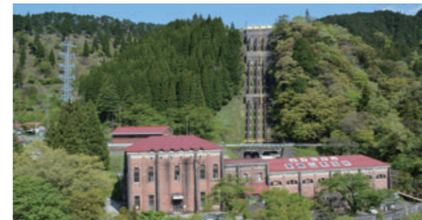
Higashi-Yokoyama Power Plant
