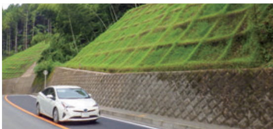
Slope constructed using the GT frame®
