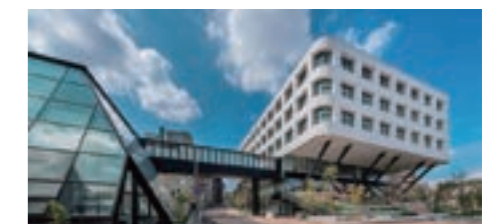
Suemori Campus, Aichi Gakuin University Clinical Education and Research Building, Tsukimizaka Terrace (Aichi Prefecture) Orderer: Aichi Gakuin University
