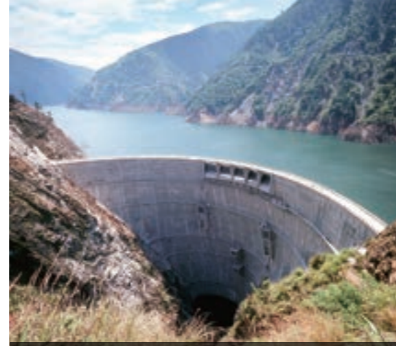
Tech (Takken) Dam
