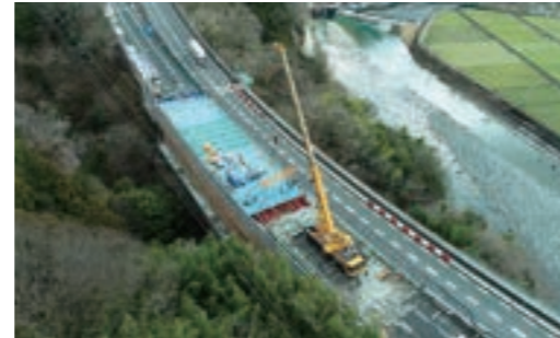
Tomei Expressway (specific renewal work) Sakawagawa 2 bridges floor slab replacement work
