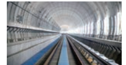
Civil engineering work for Kita-Osaka Kyuko Line extension line project (Osaka Prefecture) Customer: Kita-Osaka Kyuko Railway Co., Ltd.
