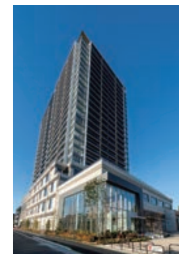
Livio Tower Hazawa Yokohama-Kokudai (Kanagawa Prefecture) Orderer: Nippon Steel Kowa Real Estate Co., Ltd. Mitsubishi Estate Residence Co., Ltd.
