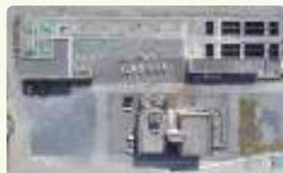
Comprehensive operation project for facility improvement at the Ofunato Sewage Treatment Plant
