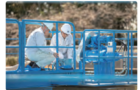
Work Scene of the Kumamoto Prefecture Ariake/Yatsushiro Industrial Waterworks Operation Project
