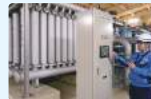
Work Scene of Water Service Kihoku's Operations
