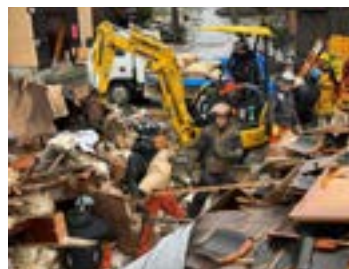
Removing debris to rebuild a damaged sake brewery
