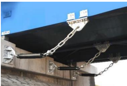
Prevention device for bridge fall③
