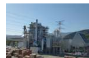
Biomass Power Plant (Ibuki Green Energy Co., Ltd.)
