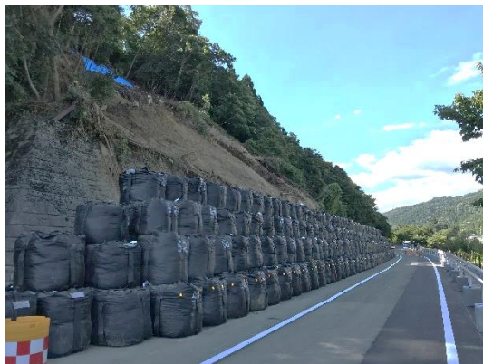
Weather-resistant, large-sized sandbag “Two-ton Bag”
