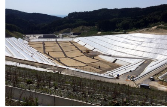
Repair work completed at disposal site
