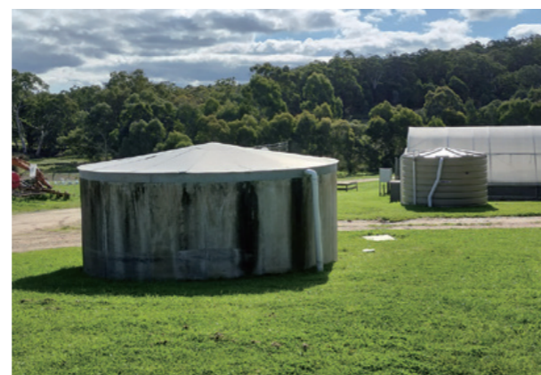
Jurlique: Flame-retardant tanks to store rainwater
