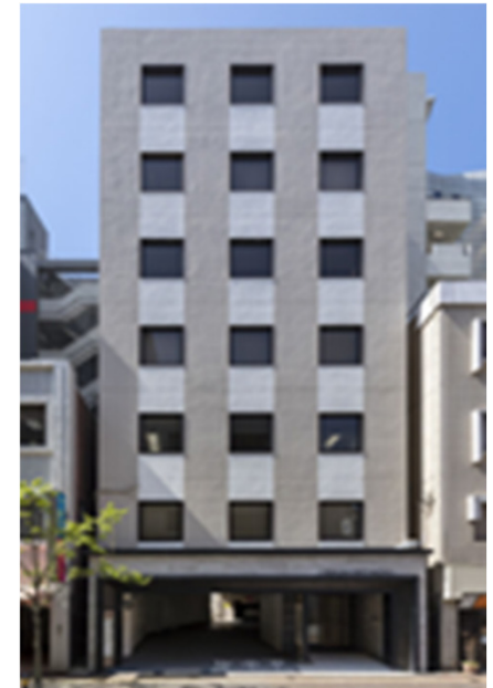
Ichigo Tenjin North Building
