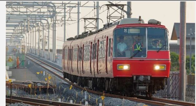
Nagoya Railroad Inuyama Line Hotei Station main line track (Konan City, Aichi Pref.)
