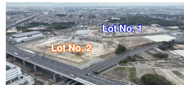
Aerial photo of the site (as of March 31, 2024)
