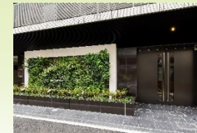
GENOVIA Higashi-Nihombashi Ekimae green veil
