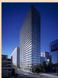
Wellith Urban Shinagawa Tower Total floor space: 16,657.11 m 2
