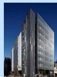
Urbannet Ginza 1-chome Building Total floor space: 11,877.63 m 2
