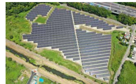
Solar power generation facility in Wakaba Ward, Chiba City
