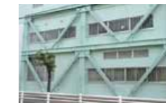
An example of reinforcement work
