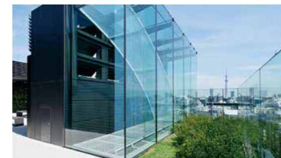
Natural ventilation (rooftop solar chimney)
