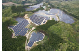
Mega solar power plant in Kawasaki Town, Miyagi Prefecture
