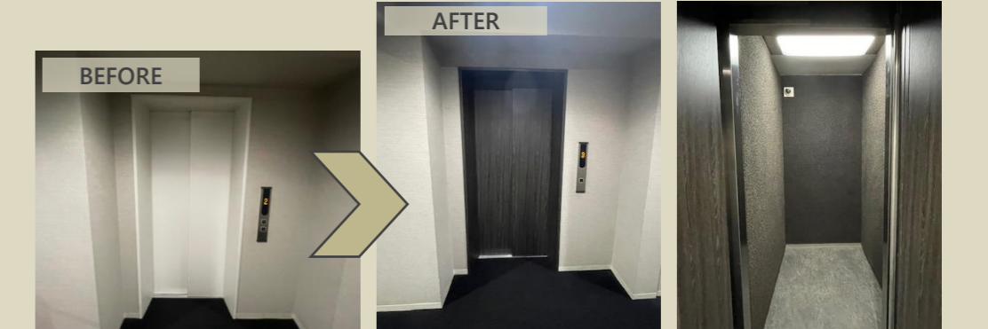
Installed interior materials that create a sense of luxury in the elevator
