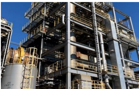
Waste incineration facility
