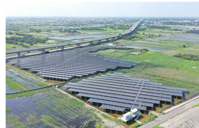
The Case Number 1 solar power plant located in Dacheng Township, Changhua County
