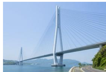
Tataro Bridge (1,480m)
