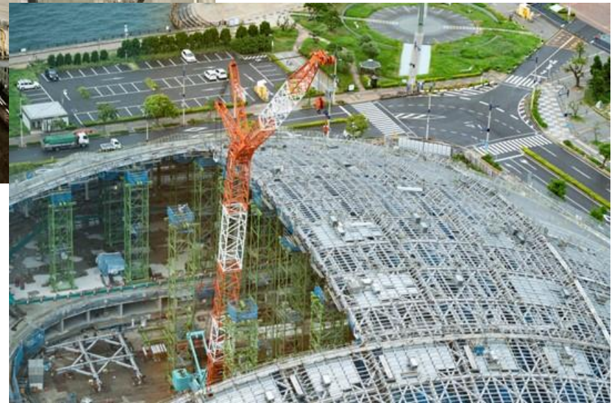
New Kagawa Prefectural Gymnasium steel construction work OBAYASHI CORPORATION and other JVs
