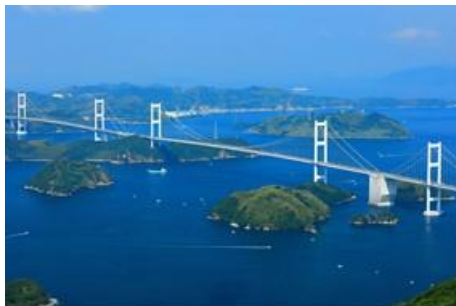
Second Kurushima-Kaikyo Bridge
