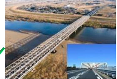
Tohoku Expressway Tone River Bridge seismic reinforcement work JV of MMB and TEKKEN CORPORATION East Nippon Expressway Company Limited
