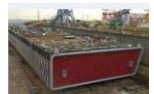
Tokyo Bay Umi-no-Mori Tunnel immersed tube tunnel
