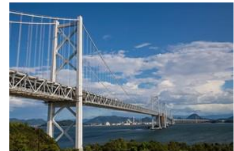
Kita Bisan-Seto Bridge and Minami Bisan-Seto Bridge
