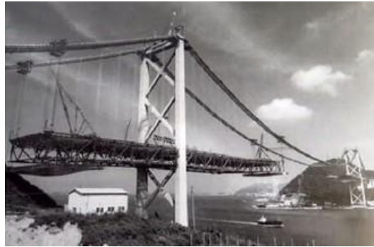
Kanmon Bridge (1,068 m)
