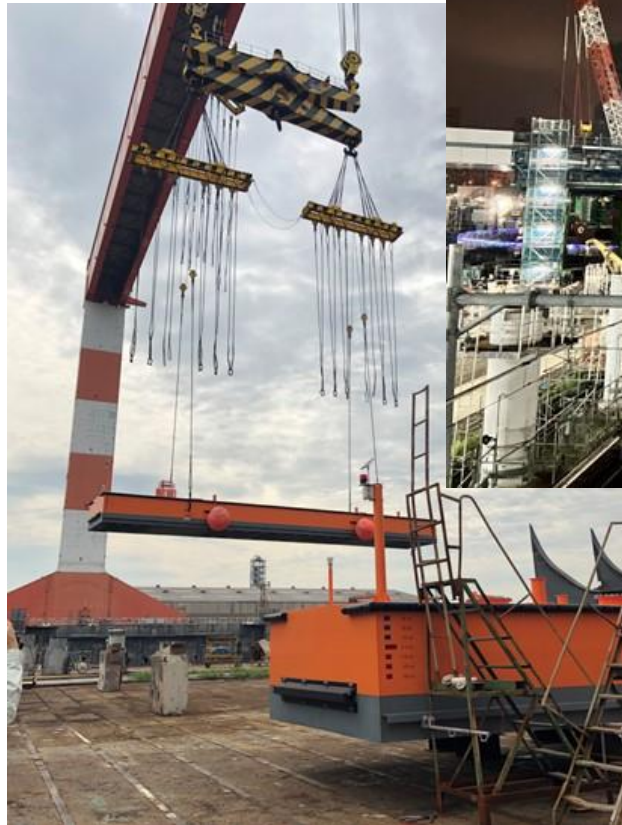
BOAT RACE EDOGAWA floating breakwater manufacturing PENTA-OCEAN CONSTRUCTION CO., LTD.
