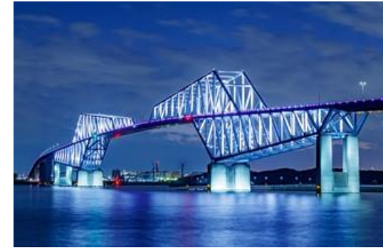
Tokyo Gate Bridge (2,618 m)
