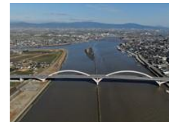
Ariake Chikugo River Bridge
