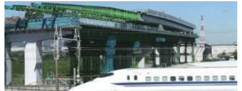
Sagami Jukan Expressway No. 16 Bridge near the Tokaido Shinkansen 50K900 point
