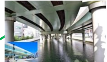
Superstructure, bridge pier, and foundation construction at a connection to a tunnel on the Inner Circular Route 6 (Nihonbashi area) Mukojima Line Industry-spanning JV of JFE, MMB, Kajima, and TOA Metropolitan Expressway Co., Ltd.
