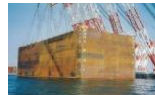
Minami Honmoku steel caisson
