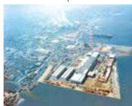
Construction of the New Mishima Mill
